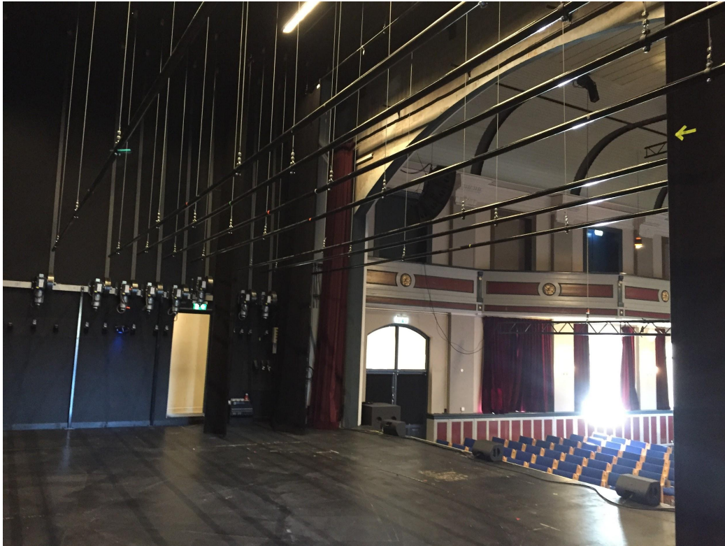
9 motorized hoists downstage
